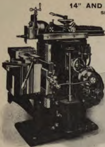
FIG. 11183. 14" SHAPER, MOTOR DRIVEN.
